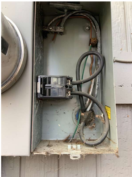
Electric Panel: Amperage 100
