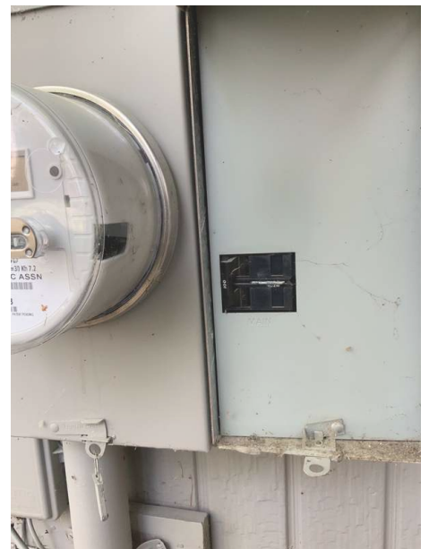
Electric Panel: Location of Main Disconnect Beside Meters
