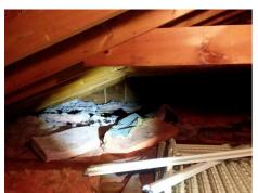
Attic Insulation: Insulation Type Attic Insulation: Depth Of Insulation 4 Inches
