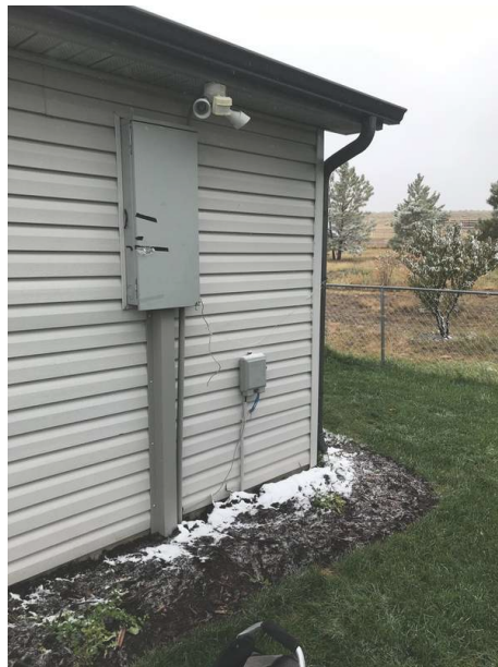
Main & Subpanels, Service & Grounding, Main Overcurrent Device: Main Panel Location Exterior
