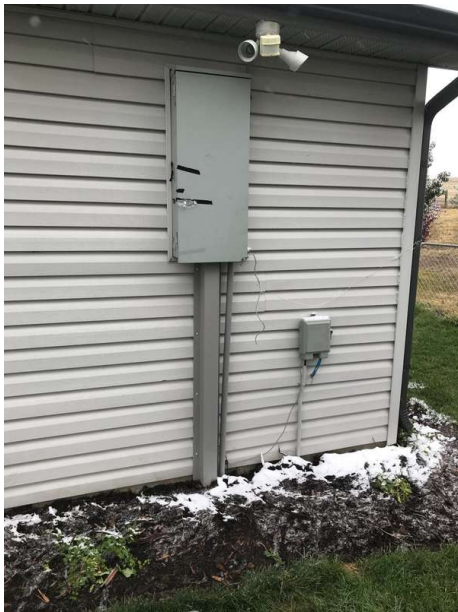
Service Entrance Conductors: Electrical Service Conductors Below Ground
