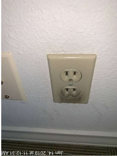
Overheated Receptacle.
