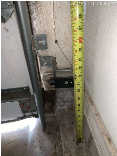
Garage door sensors are installed higher than six inches.
