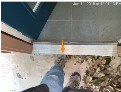
Threshold overhang is a trip hazard.
