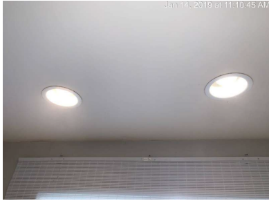
Recess lighting not rated for use in a wet location.
