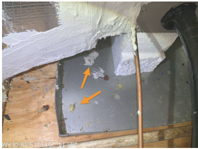
Debris in condensate pan should be cleaned.
