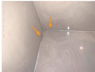
Seal master bathroom bench.
