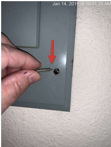
Sharp screws used to install panel cover.
