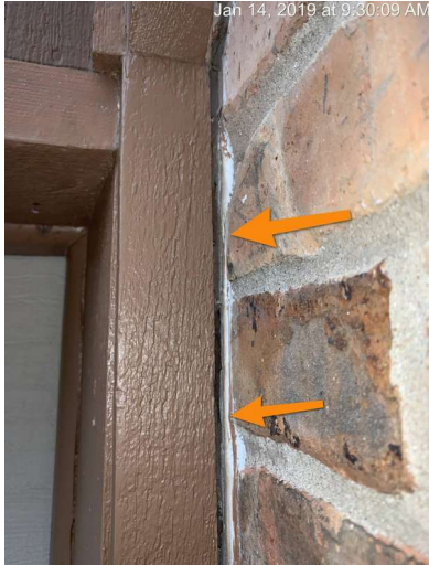
Seal to prevent water intrusion.
