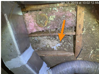
Missing attic insulation.
