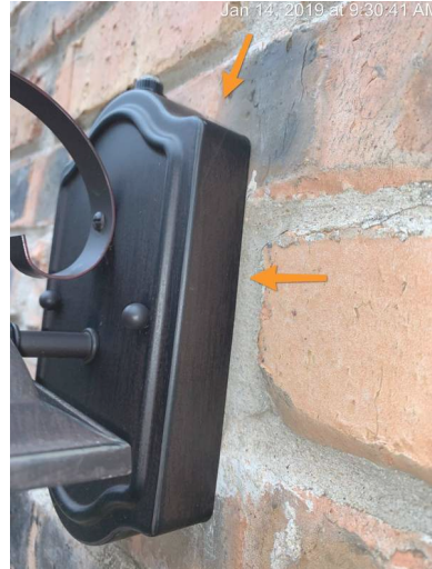
Seal to prevent water intrusion.
