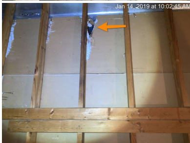
Opening in draft stop
