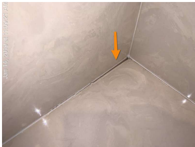
Seal master bathroom bench.
