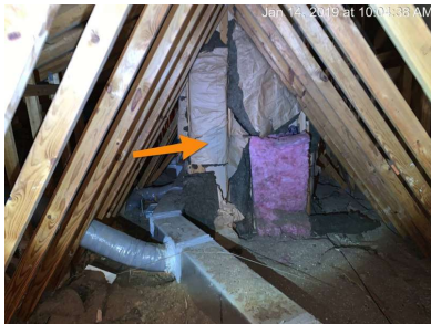
Vertical insulation attached to skylight.
