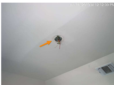
Fixture missing leaving exposed wiring.
