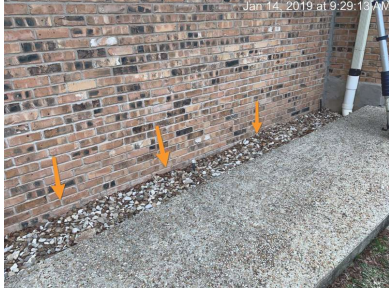
Should be 4-6' inches of foundation visible.
