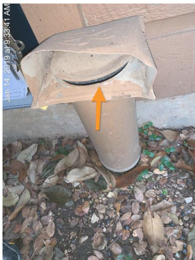
Flapper on dryer vent not closing. Recommend replacement.
