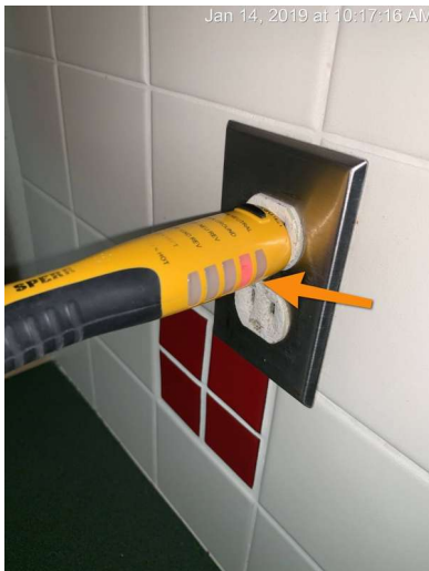
Receptacle showing "open ground"
