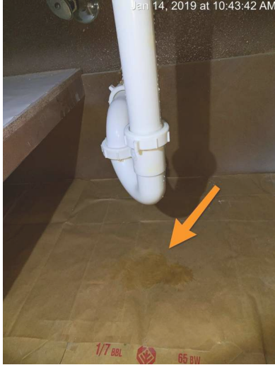
Bar sink leaking.
