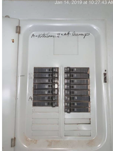
Sub-panel with cover.
