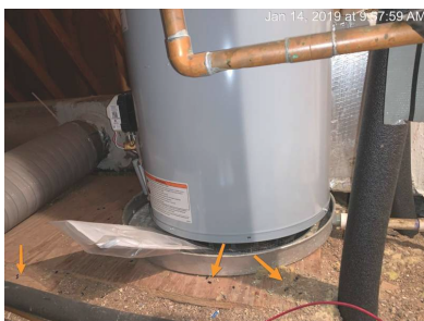
Evidence of rodent activity.
