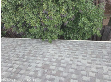
Cut tree limbs back a minimum of three feet from roof covering.
