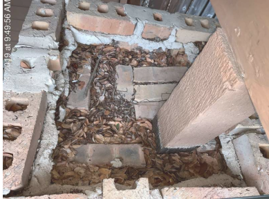
No cap for brick column.
