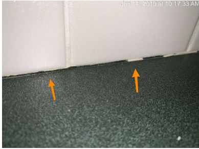
Seal kitchen back splash to prevent moisture intrusion.
