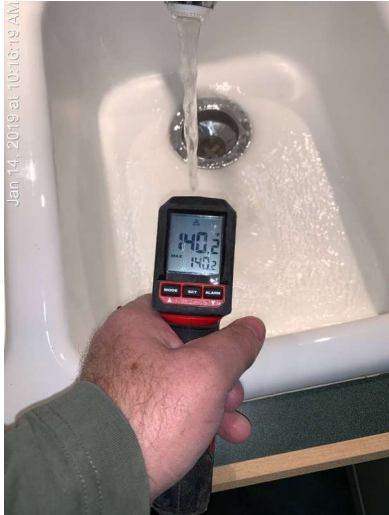
Water temp 140 at kitchen sink.
