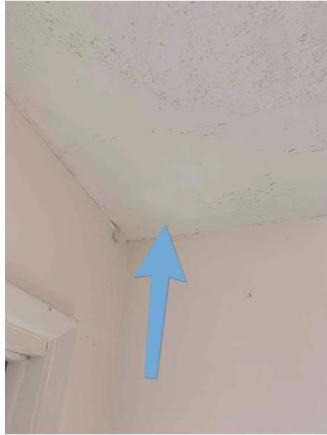
Back storage room
