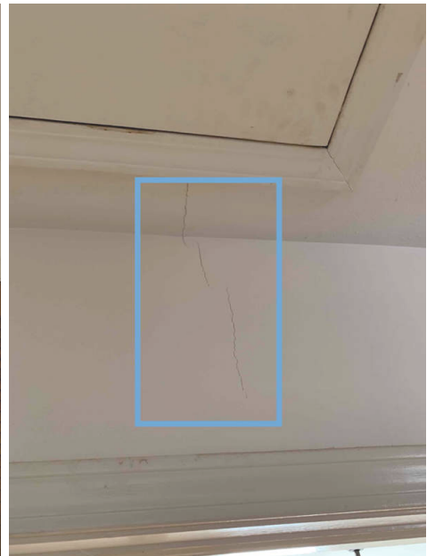
Front hallway by attic access
