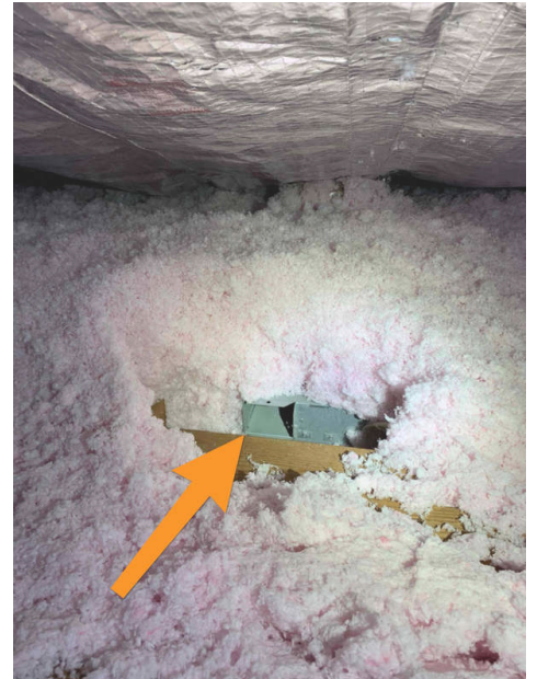
Guest Bathroom Front part of home
