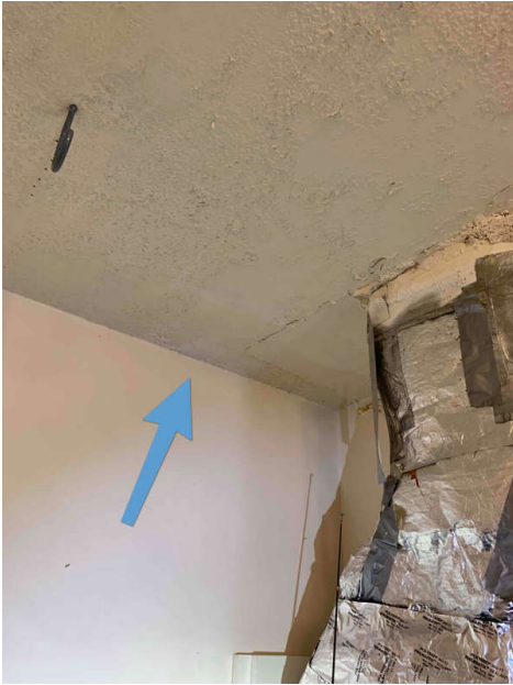
Back storage room
