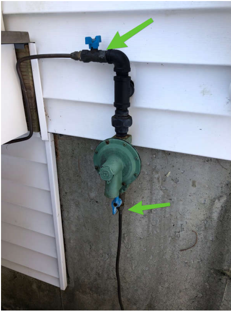
Exterior gas shutoffs
