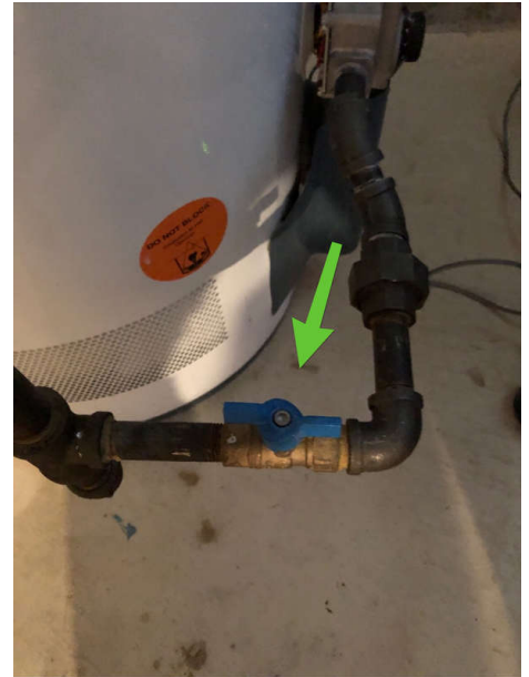
Gas Shut Off
