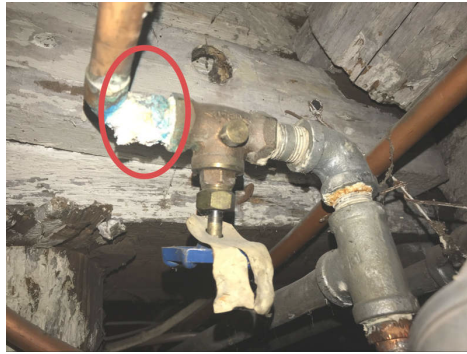
Above Water Heater
