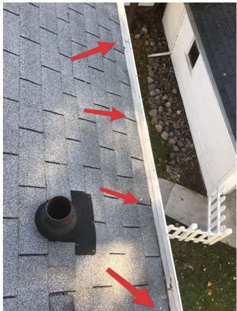
West Side-Entire Bottom Course
