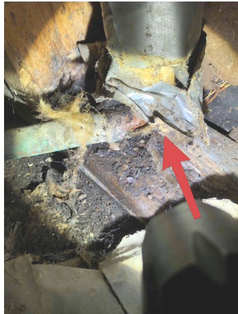
Wet/leaking hit wster pipe Garage
