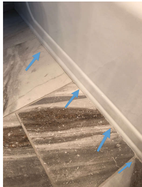
2nd floor Hall Bathroom
