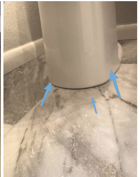
2nd floor Hall Bathroom
