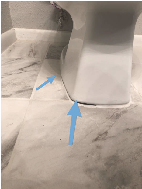
1st Floor Bathroom
