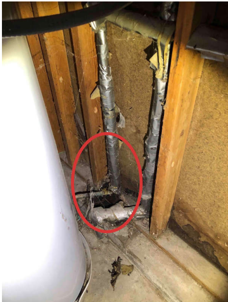
Hot water pipe Garage
