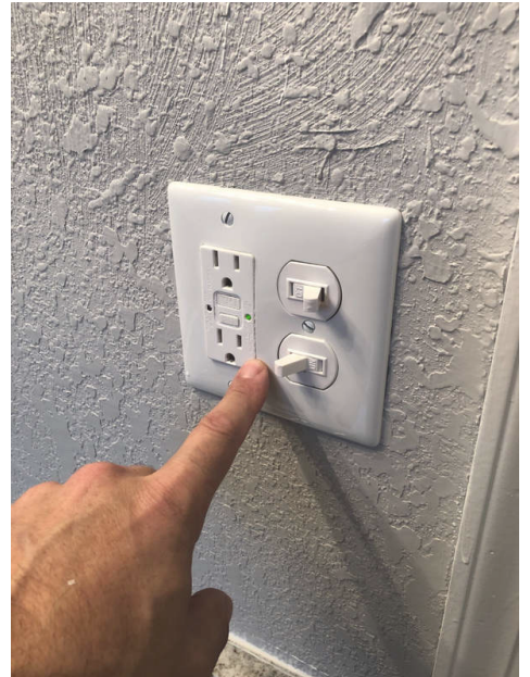
2nd floor Hall Bathroom
