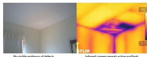
No visible evidence of defects
