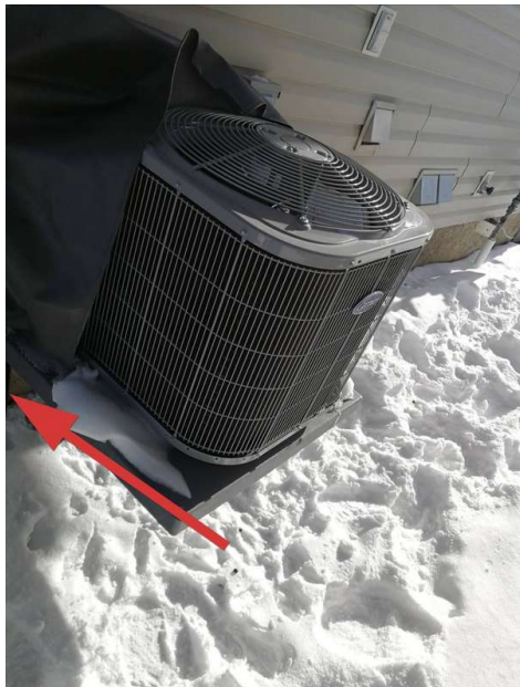
Ac unit attached to the foundation.
