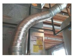
**Distribution Systems: Ductwork** Non-insulated
