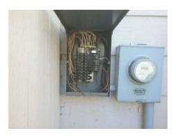
Main & Subpanels, Service & **Grounding, Main Overcurrent Device: Panel Capacity** 100 AMP
