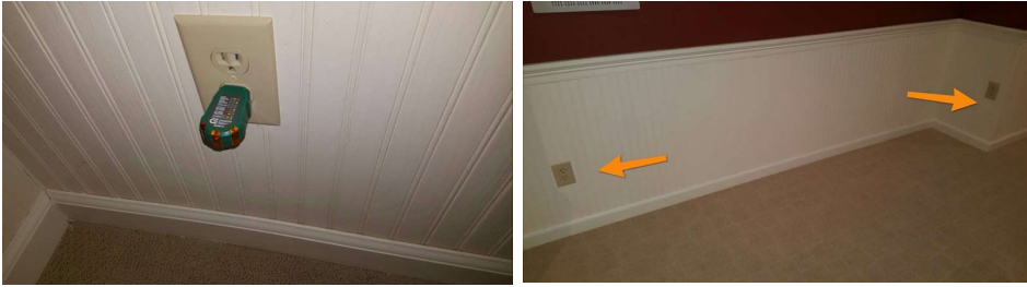
2 receptacles in the basement are affected.
