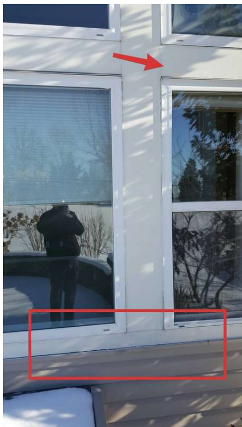
The only visible and accessible area was completely rotted away. The rest of the wall could not be evaluated.
