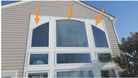
Rear Left. There is no flashing installed at the rounded windows at the top.
