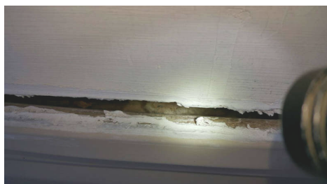
Wall sheathing is completely rotted away and the insulation is visible
