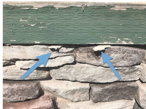
South (Mortar Deterioration)
