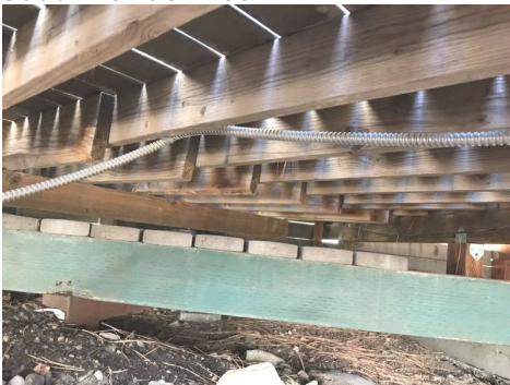
South - Under Deck
