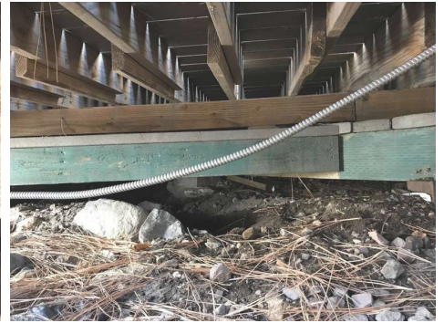
South - Under Deck
