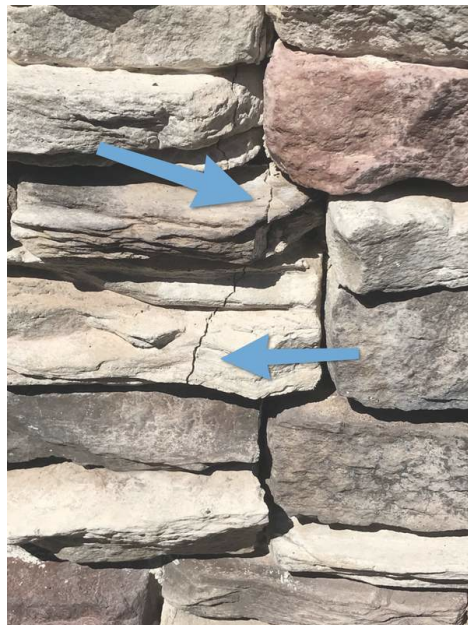
South (Stress Crack)
