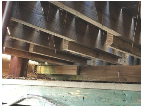
South - Under Deck
