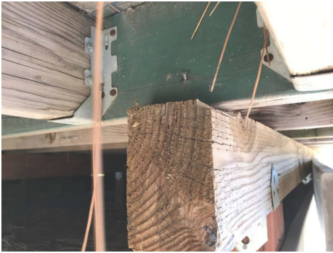
South - Under Deck
