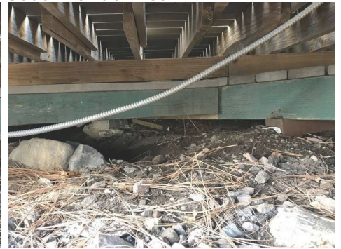
South - Under Deck
