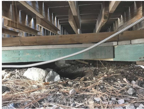
South - Under Deck
