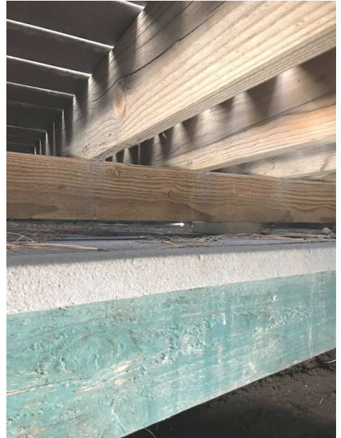
South - Under Deck
