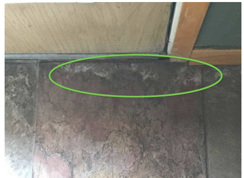
Exterior South Utility/Laundry Room
