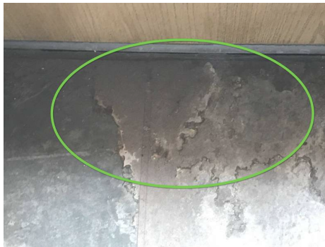
Exterior South Utility/Laundry Room
