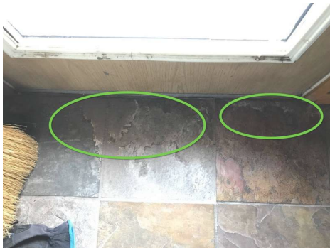
Exterior South Utility/Laundry Room
