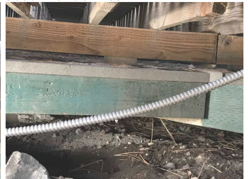
South - Under Deck
