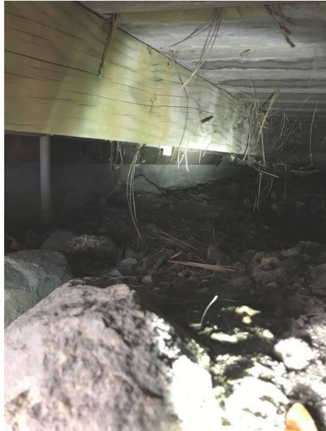
South - Under Deck
