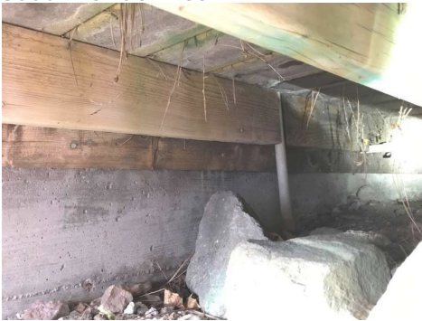
South - Under Deck
