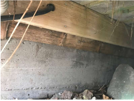
South - Under Deck
