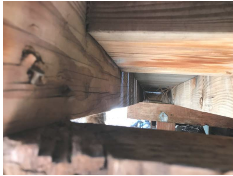
South - Under Deck
