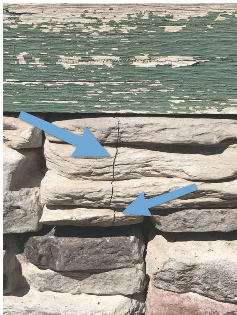
South (Stress Crack)
