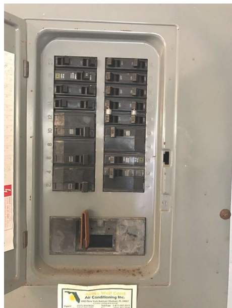
Service and Grounding Equipment, Main Overcurrent Device, Main and Distribution Panels 2: Main Panel Overcurrent Protection 150 Amp
