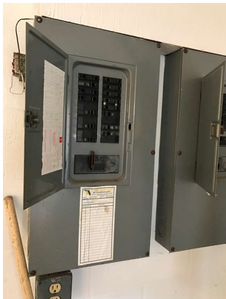
Service and Grounding Equipment, Main Overcurrent Device, Main and Distribution Panels 1: Main Panel Location Garage
