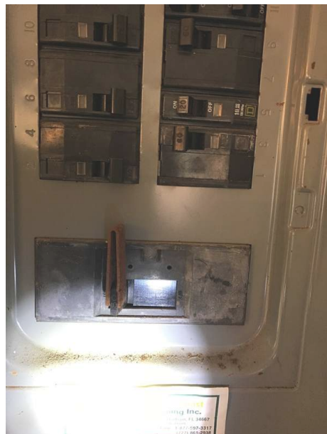
Service and Grounding Equipment, Main Overcurrent Device, Main and Distribution Panels 1: Main Panel Rating 150
