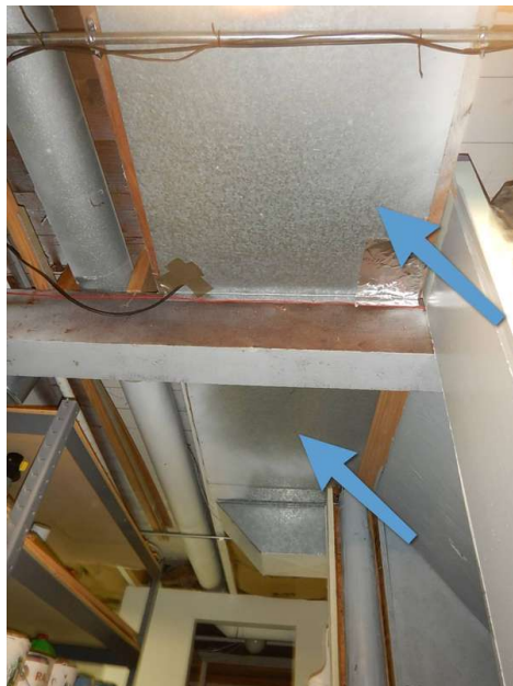
using building cavities as return plenums results in significant duct leakage - difficult to seal and clean
