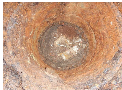
basin is heavily corroded, full of debris, and inspector unable to verify if there is a drain at bottom of basin, or where it may be plumbed to - further evaluation is recommended
