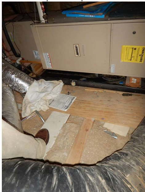
installed pathway and service platform are inadequate and pose a hazard
