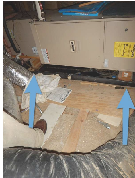
furnace rests on ceiling framing
