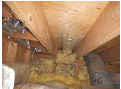
soffit vents with installed chutes
