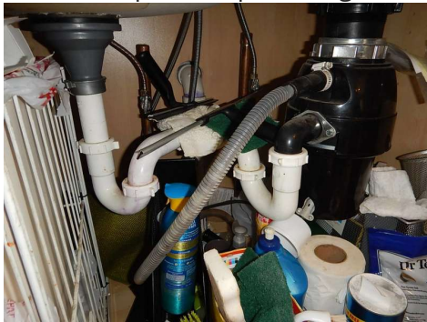
High Loop installation - IL prohibits connections to disposers
