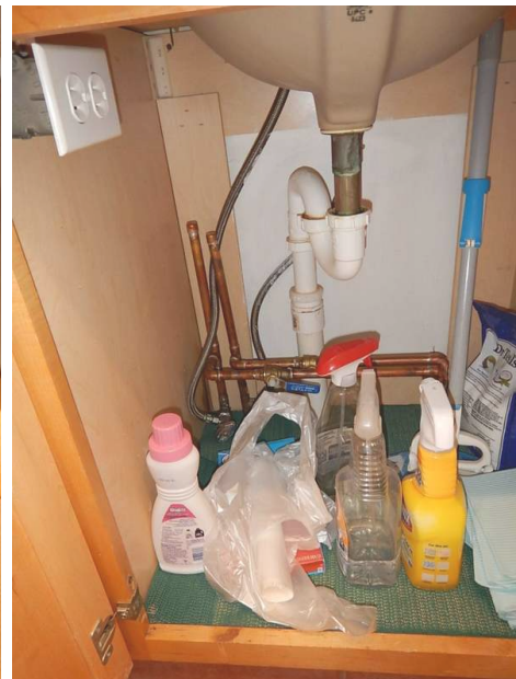
2nd Floor Bathroom
