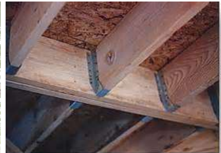
Joist Hangers
