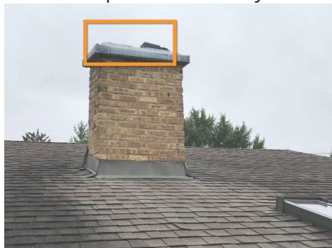
Fireplace flue appears to have no spark arrestor
