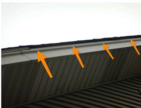
missing section of rake edge flashing
