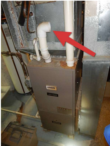
melted and scorched plastic bushing near water heater draft hood, indicative of back drafting condition
