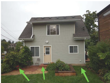
negative grading @ East side of home
