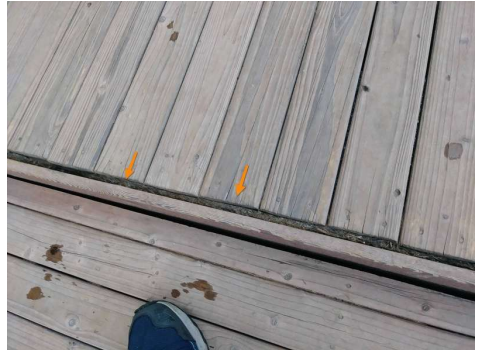
Debris is filled in-between the deck and fascia board.
