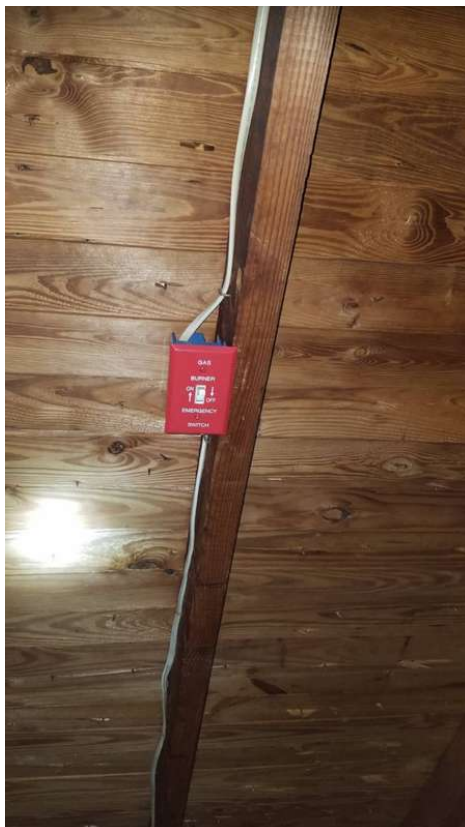
Emergency Shut Off of attic Furnace.
