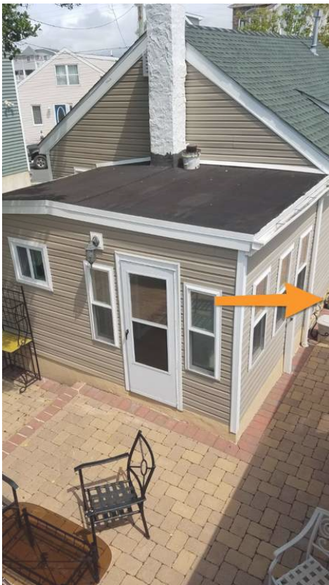
Gas meter location in driveway.
