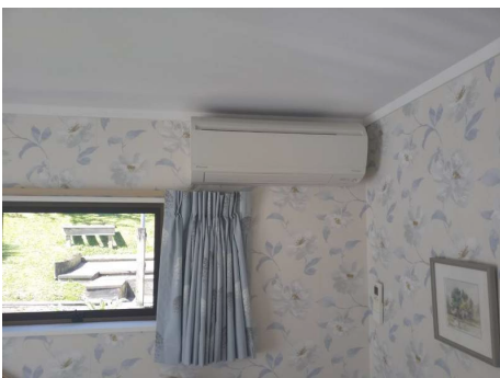
Electrical and Heating: Heating type and operation inspected Heatpump
