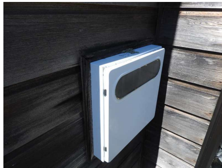
Inspected presence of : Electricity services
