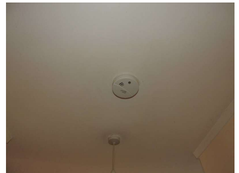
Inspected presence of : Fire warning and control systems (including smoke detectors)
