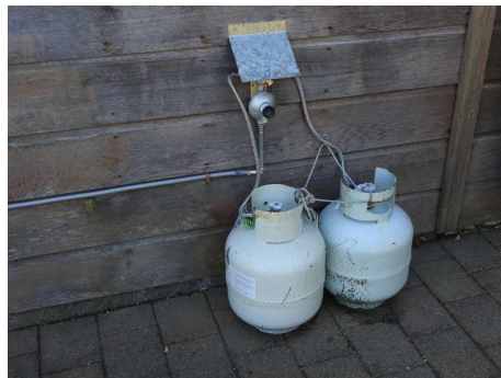
Inspected presence of : Gas services
