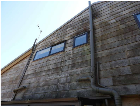
Door - Aluminium units: Joinery Inspected Safety glass, Double glazing
