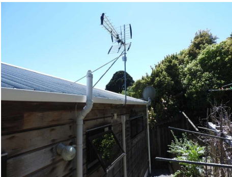
Inspected presence of : Aerials and antennae
