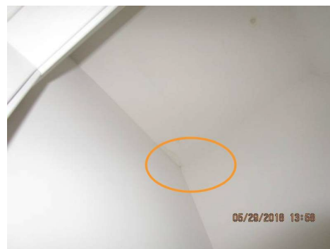
upper corner in closet
