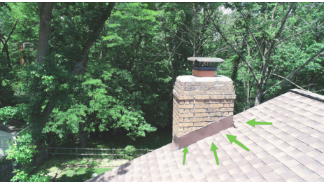
Proper Flashing Around Chimney
