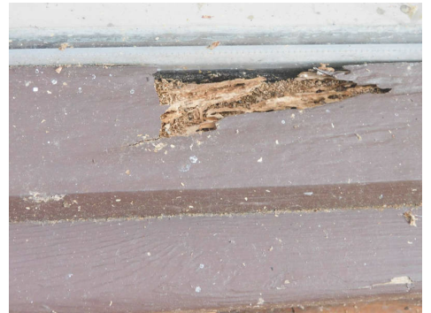
Rear of Home along Deck at Windows
