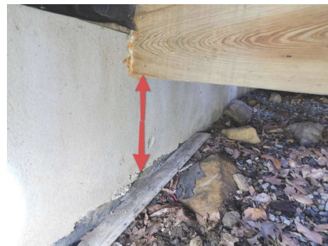
Missing Post Under Support Beam on Deck
