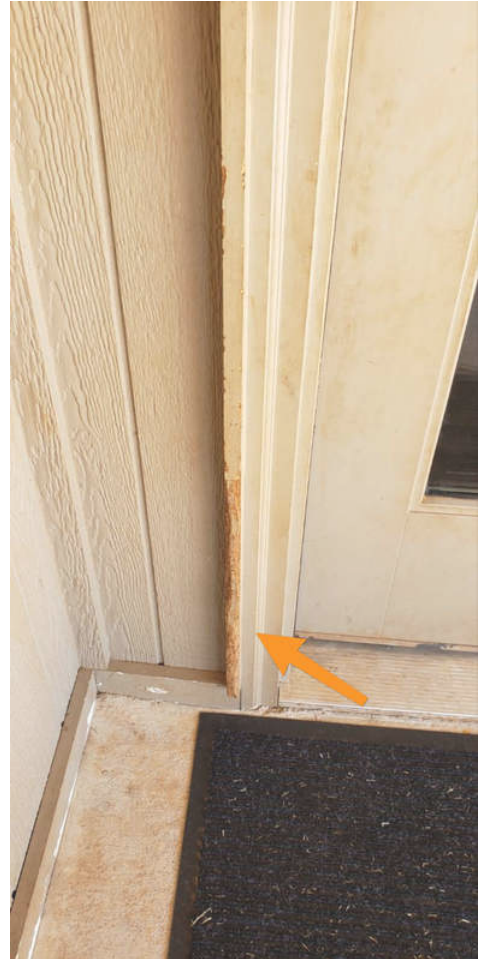
Rear Entry. Apparant dog scratches
