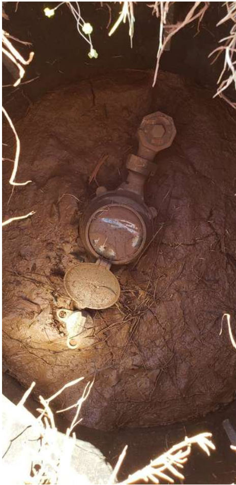
Sewage & Drain, Waste, & Vent (DWV) Systems: Plumbing Clean-Out Location Front Yard, Under Kitchen Sink
