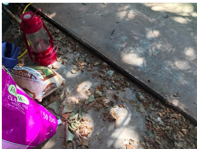
Settling garage slab
