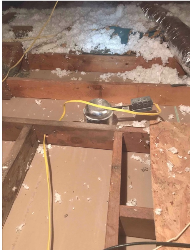
This photo was taken above the bathroom next to the garage.
