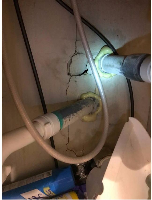
This crack was observed under the kitchen sink.
