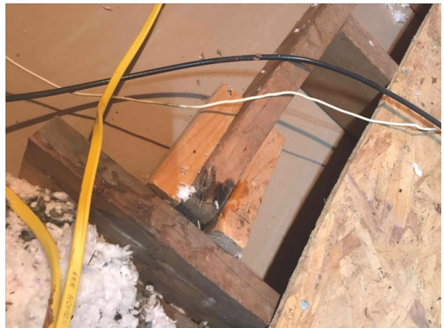
Condensation dripping on framing members.
