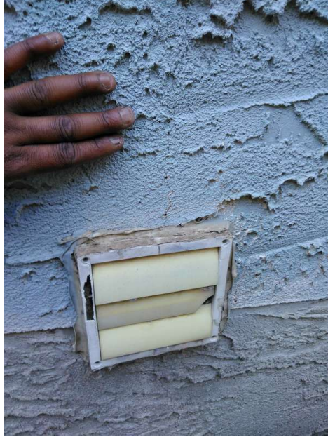
Damage replace recommended
