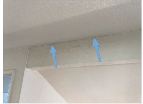
2nd Floor Hallway
