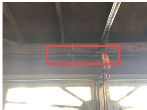
Garage Right Side
