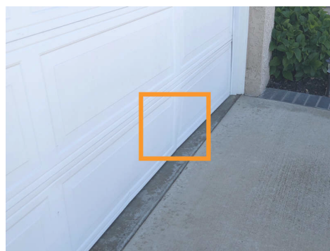
Garage Right Side
