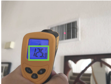
Heating Supply Temp
