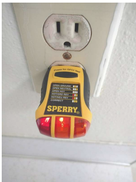
First Floor North Bathroom
