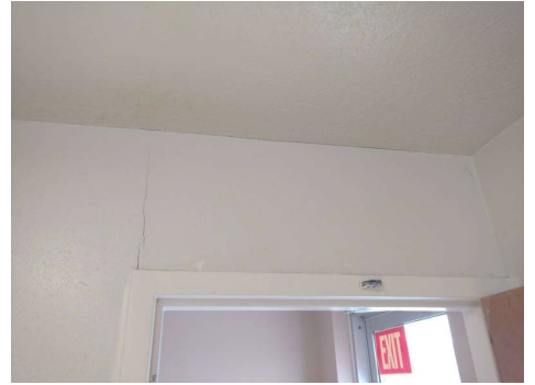
Second floor north bathroom
