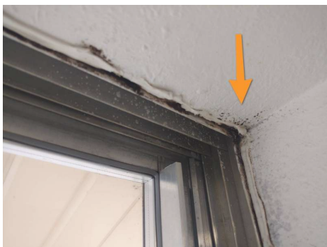
Mold observed around the window in the south bathroom on the second floor. Installing ventilation fans helps mitigate the risk of mold growth in bathrooms.
