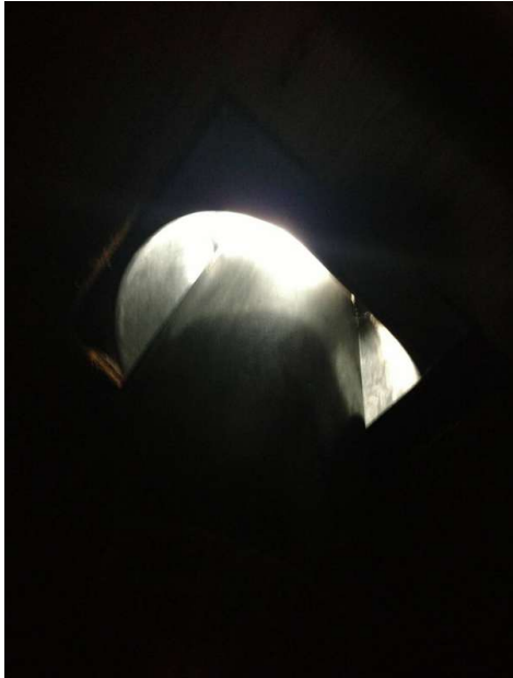
Daylight coming in from around vent pipe.
