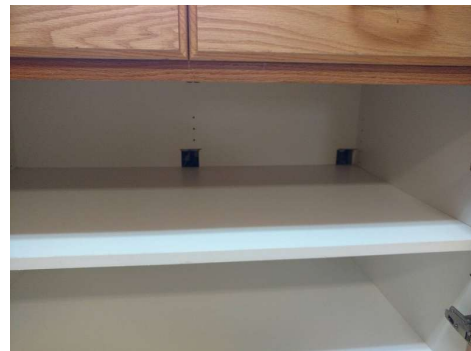
West wall in second floor kitchen.
