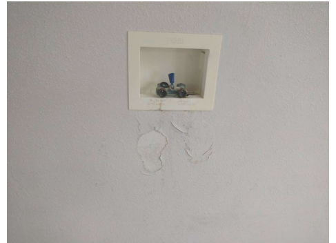
Second floor north dorm.
