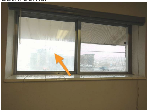
Moisture inside of the window.
