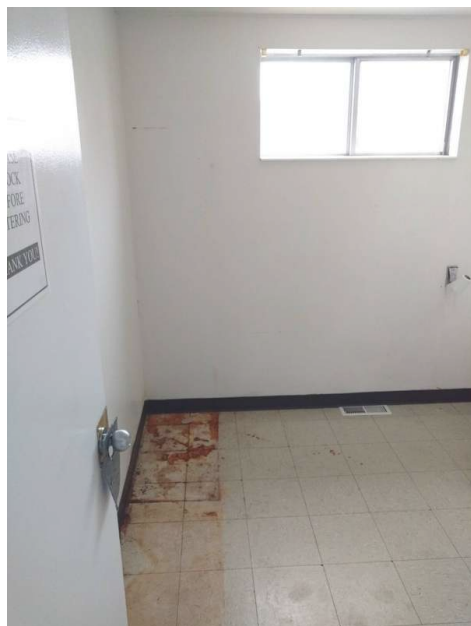
First floor north bathroom
