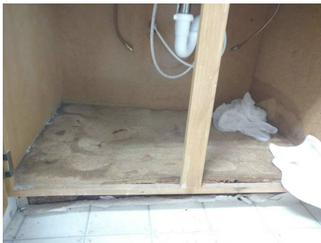
North bathroom on the second floor shows signs of water damage. No leaks were observed during the inspection.
