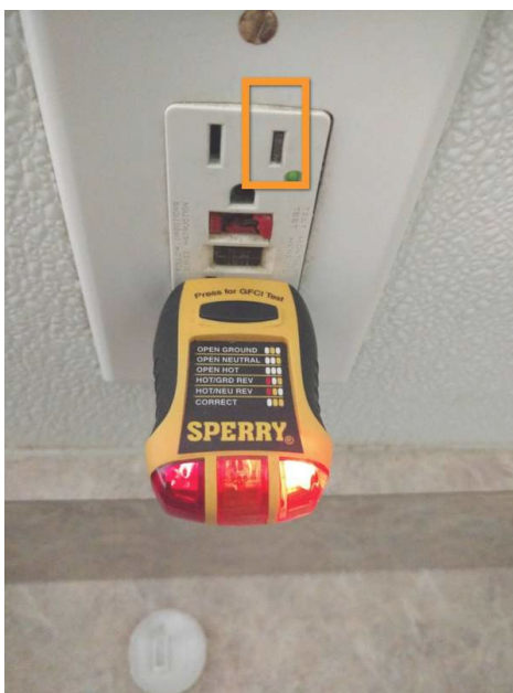
First Floor South Bathroom Top right outlet slot is blocked by a piece of an outlet protector that broke off inside. GFCI Test/Reset button broken.
