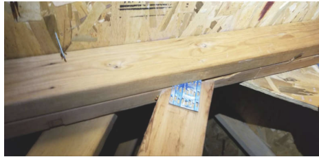
Other side of broken member
