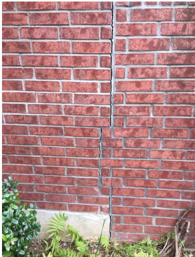
Right rear of house.
