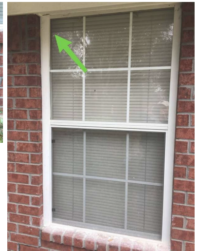
A trim piece has been added, presumably to cover a gap between the window and the brick.
