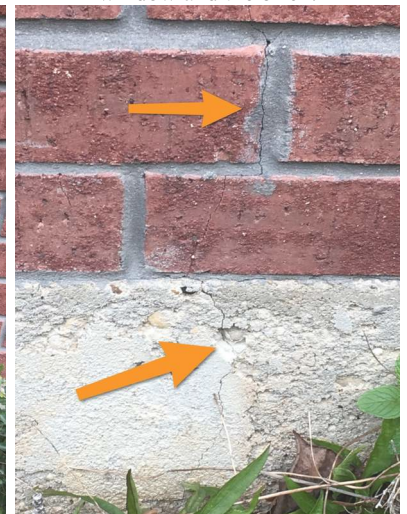
Cracks at the foundation wall and brick wall.
