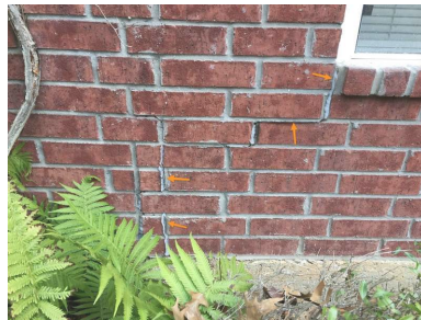
There appears to be rotation of the brick face just below the corner of the window.
