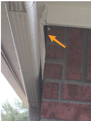
Separation of the brick mold from the wall.
