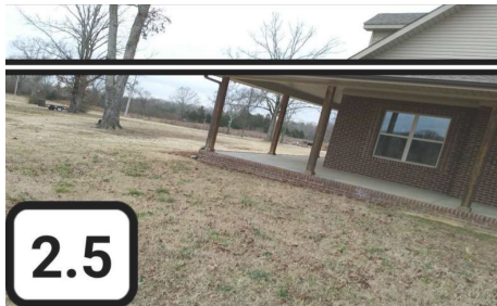
Approximately 2.5/12 roof slope. Very shallow for asphalt roof coverings
