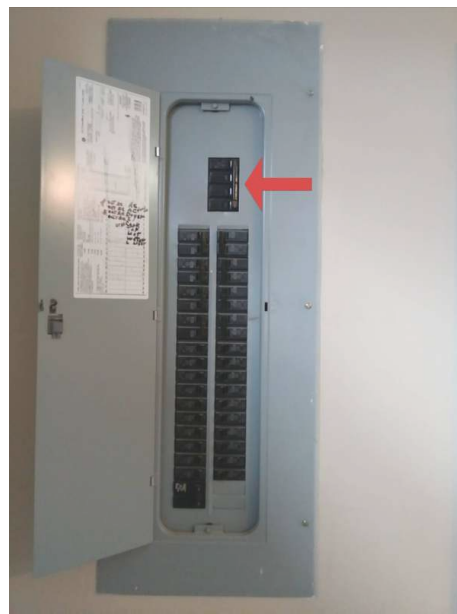
Main shut off breaker.
