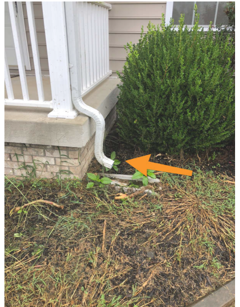
North Side Porch
