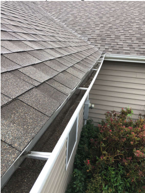
Standing water Southeast
