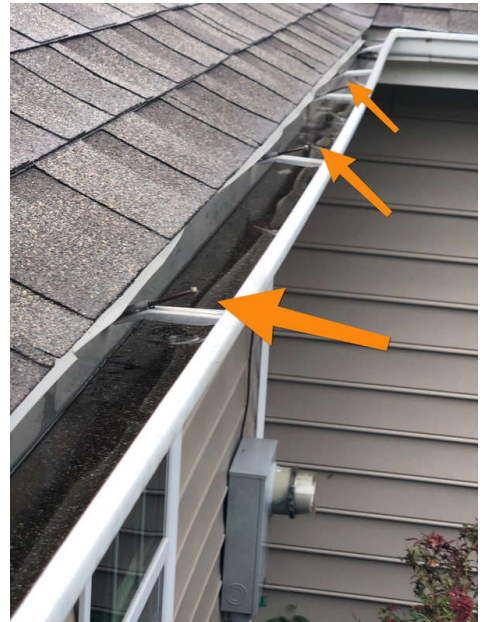
Three screws not completely installed Southeast
