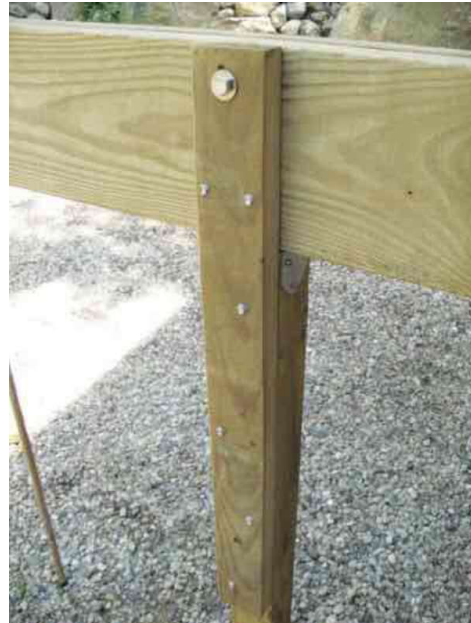
Example photo of a recommended repair for the improper post to beam connections
