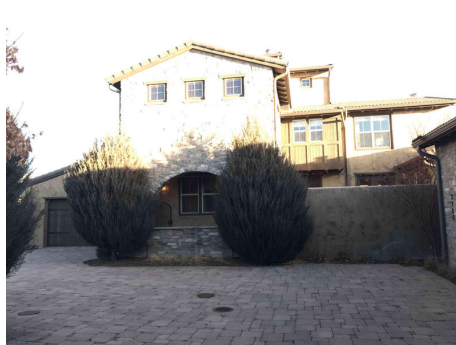
Orientation: South Exterior
