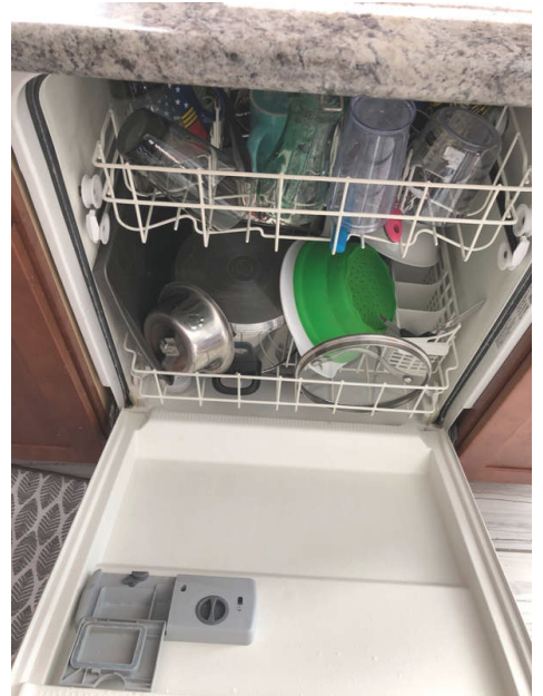
DW not attached to cabinets
