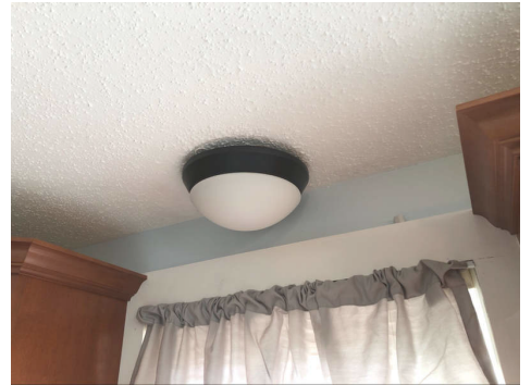
Kitchen sink light (also loose)
