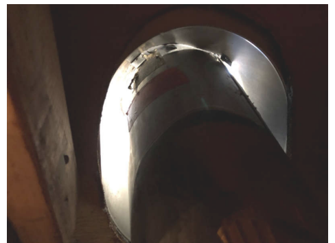
Furnace vent needs exterior flashing
