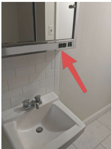
Bathroom 3rd Floor
