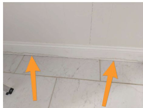
Bathroom 3rd Floor
