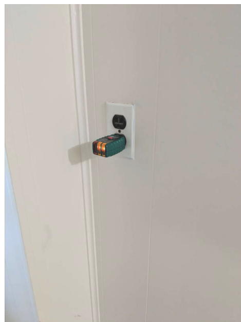
3rd Floor Bathroom
