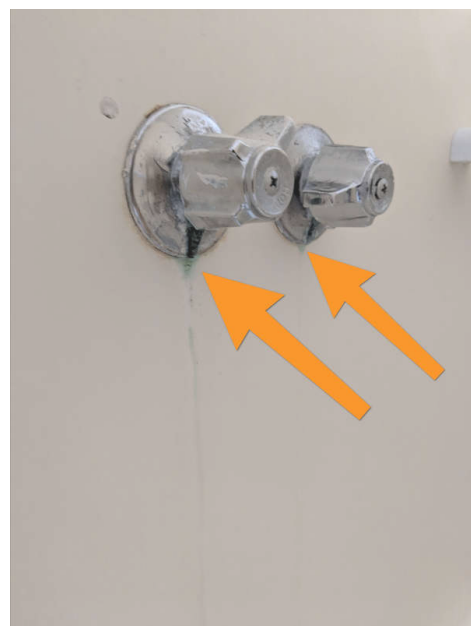
Bathroom 3rd Floor shower
