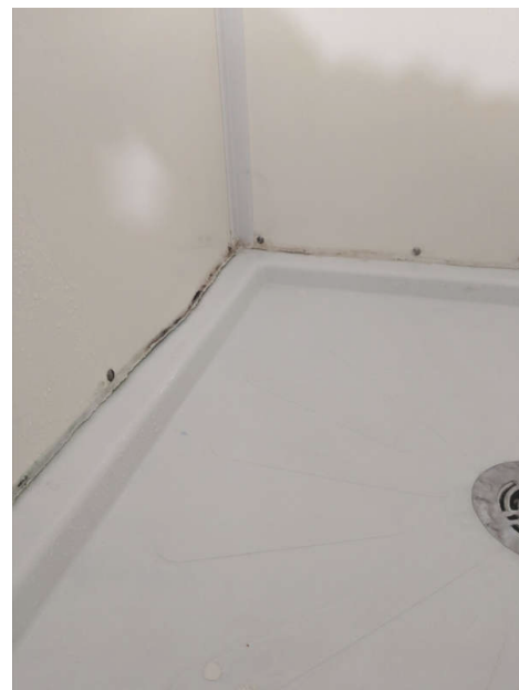
Bathroom 3rd Floor
