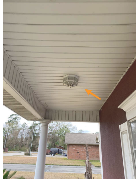
Front of House Garage
