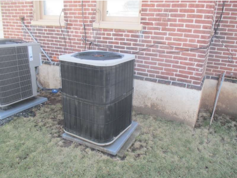
3.5-ton unit manufactured 7/98 Budget for replacement
