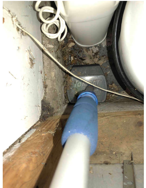
Trap observed in garage.
