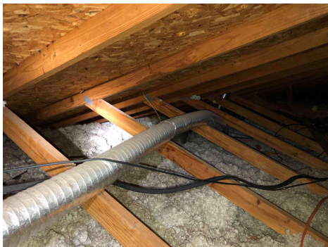
Mylar dryer duct also observed in attic.
