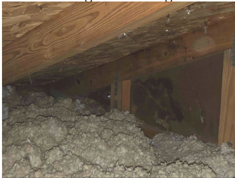
NE corner of attic.
