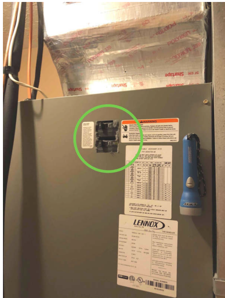
Electrical kill switch (breakers) for furnace.
