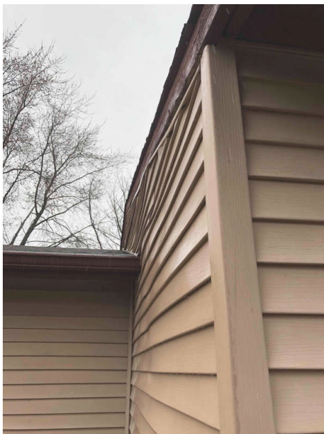
Bowing siding may be due to water intrusion.
