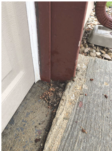
Wood trim can pull moisture from contact with concrete.
