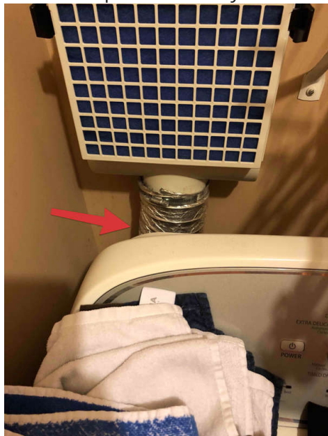
Mylar dryer duct also observed in attic.
