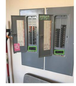
**Panel Manufacturer** Square D Panel Type / Capacity Breakers, 200 amp Service Panel Grounding Conductor Present
