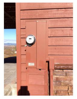
Main & Subpanels, Service & Grounding, Main Overcurrent Device: Panel Manufacturer Siemens Main & Subpanels, Service & Grounding, Main Overcurrent Device: Panel Type Circuit Breaker Main & Subpanels, Service & Grounding, Main Overcurrent Device: Panel Capacity 200 AMP
