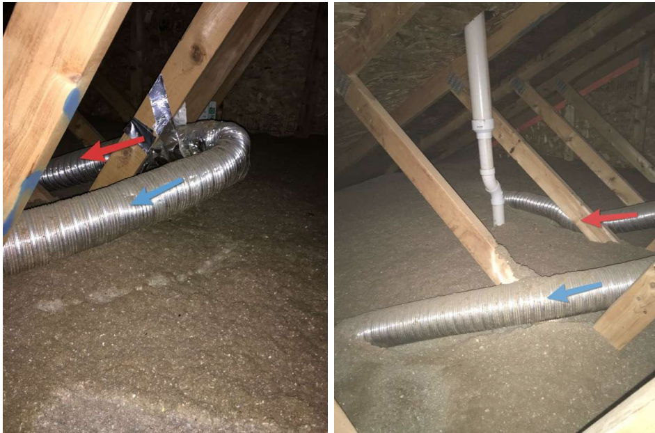
Red To Master Bath : Blue to Second Floor Main
