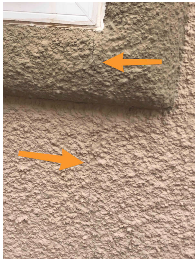
West side of home
