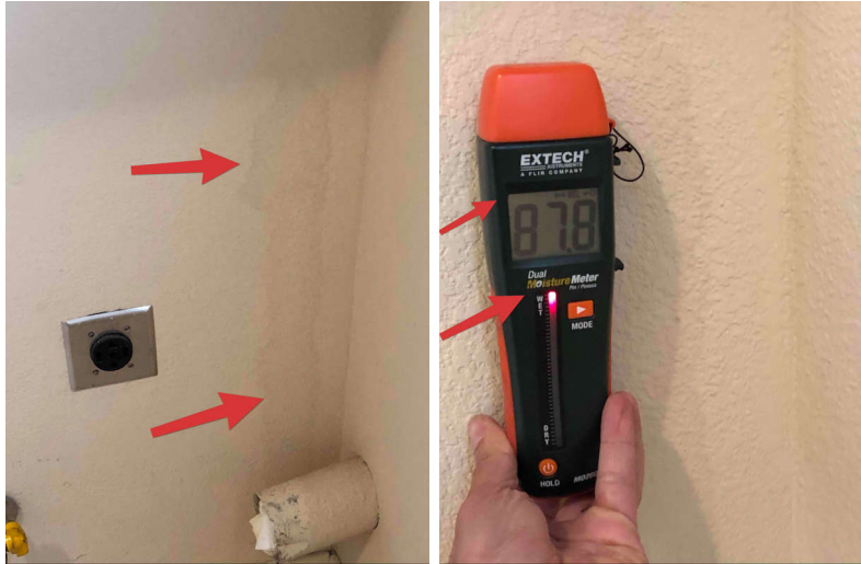
Moisture meter reading
