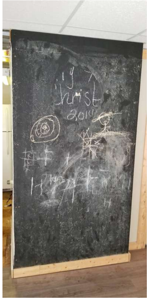
Chalkboard panel must be removed to access light switch as well as the HVAC air handler and water heater.
