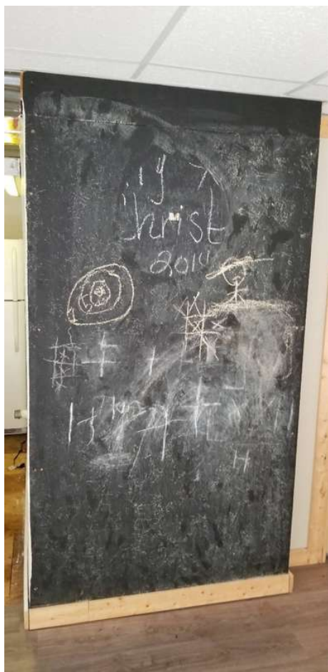
The water heater as well as the HVAC air handler are located behind this chalkboard panel
