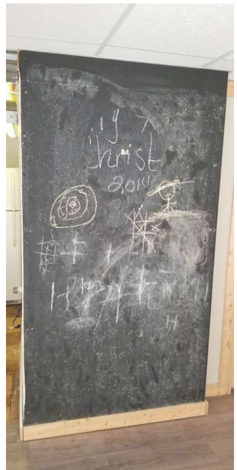
HVAC air handler and water heater located behind chalkboard panel
