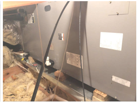
Air handler unit
