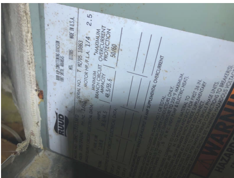
Air handler unit label. Manufactured in 2005.
