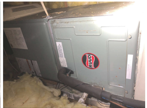
Air handler unit
