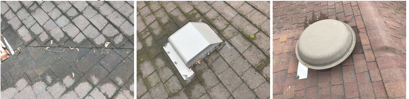
The valley flashing is cracked and worn.
