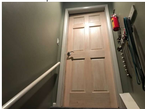
There is no 3-way switch to the basement
