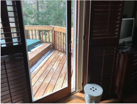
Bedroom door does not lock
