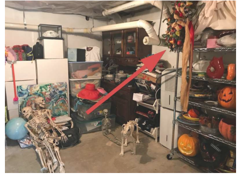
Duct tape is used on the connection where the pipe leaves the building.
