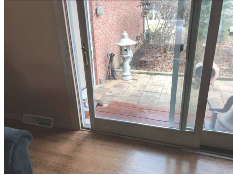
Family room door does not lock
