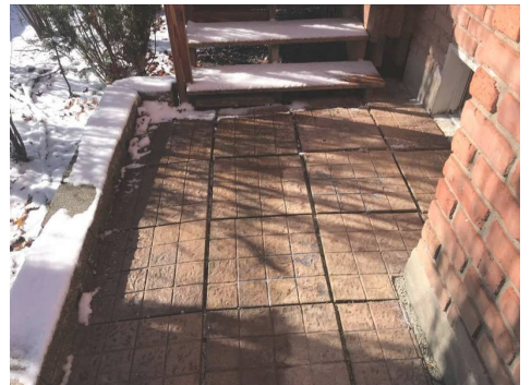
The patio settled on the left side.
