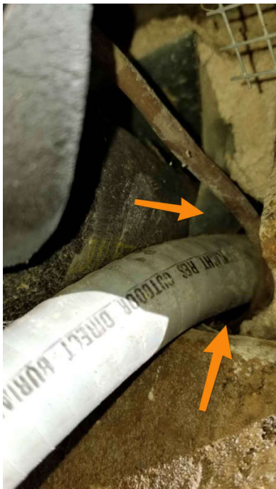
Air Conditioner Lines
