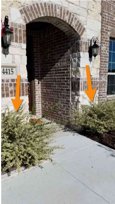
Front Porch Area
