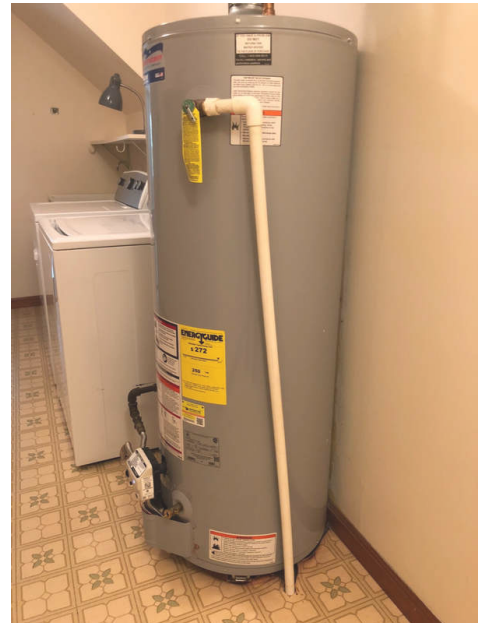
Incorrect TPR Valve
