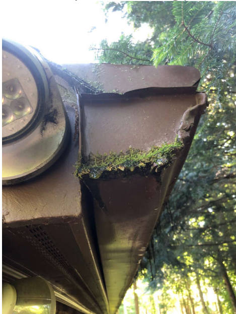
Moss Growing In Leak
