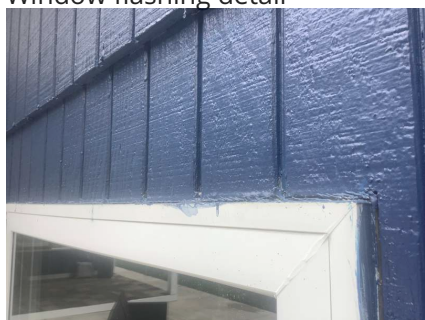
Window flashing detail
