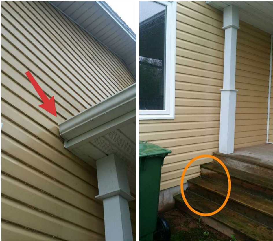
Water over flowing gutter landing on porch steps due to missing Kickout Flaxhing
