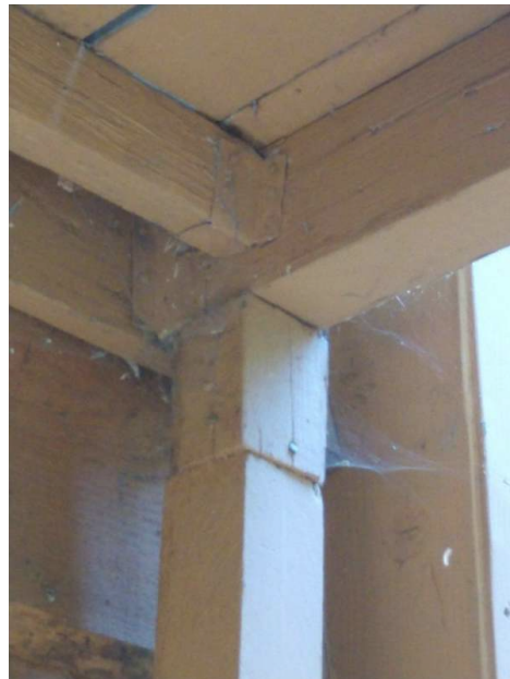
An extension was added to this post supporting the load of a deck.
