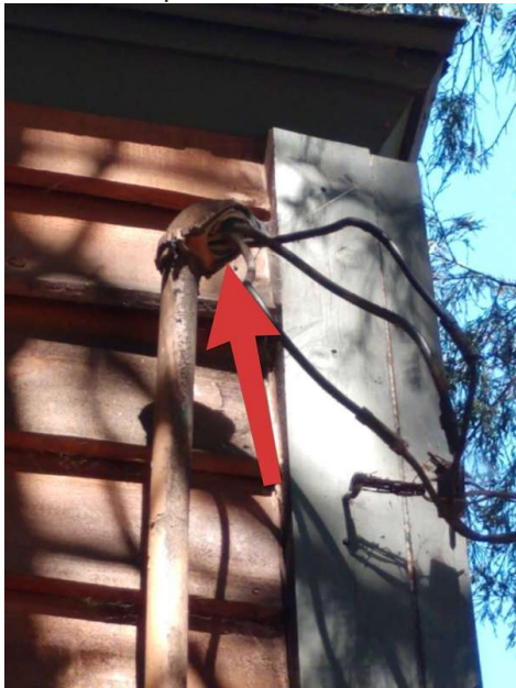
Plastic protective insert is missing.
