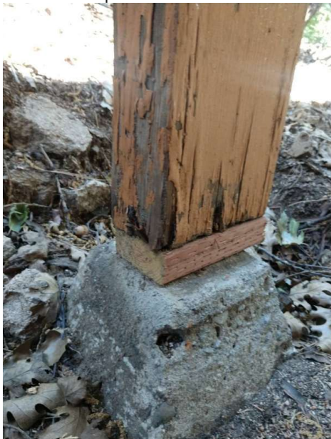
No mechanical fastener securing base to post.
