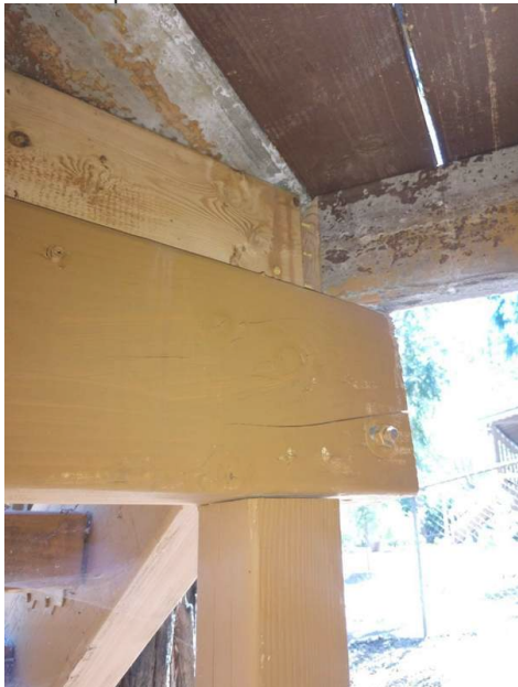
The post to beam connection should be in a bracket that provides a more secure attachment. The stair stringers should be mechanically fastened by use of a bracket, lag or machine bolts.
