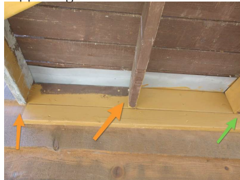
Orange arrows indicate unsupported deck joists. The green arrow indicates a supported deck joist.
