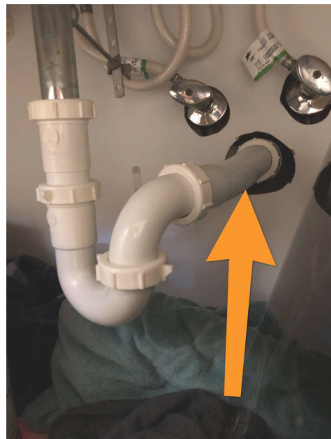
Hall Bathroom sink
