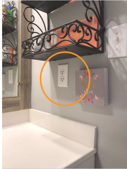
Basement hall Bathroom
