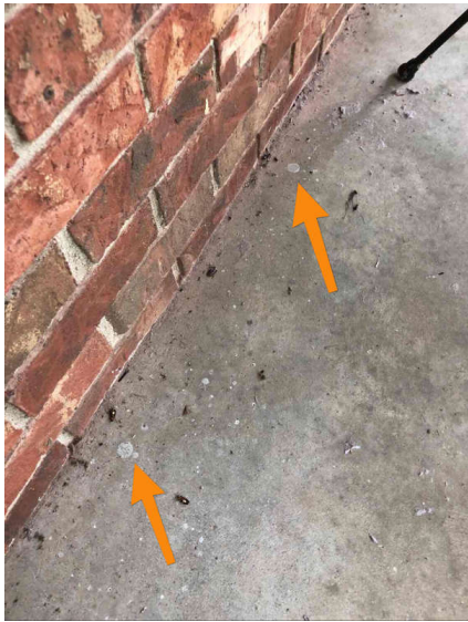
Drill holes- South patio
